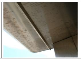
Above is detail of a canopy above a stainless steel revolving door after four years in service in the vicinity of sea water. You can see all kinds of rusty spots also known as tea stains. This is the work of aerosols, together with dirt deposits.
